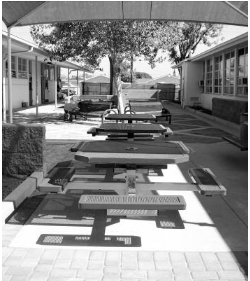
View from the west end of the newly completed Social Courtyard on the SLDC campus.
