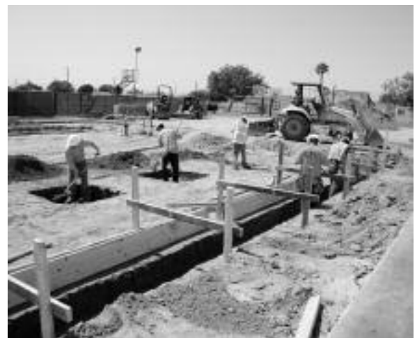
Beginning the preparation for concrete footings!
